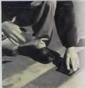
NJDOT participated in the development of a snowplowable raised reflective pavement marker. (1967)
